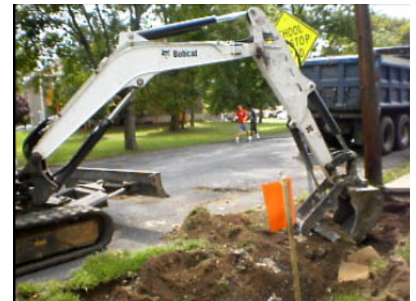
Above (top to bottom): Aerial of Walden's WWTP, Walden's new DPW Garage and workers replacing sidewalks along Wait Street in the Village.
