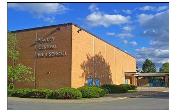
Above (top to bottom): Walden Elementary School on Orchard Street, Most Precious Blood School and Valley Central High School, in the Town of Montgomery. It is critically important that Walden retain an elementary school within the Village limits.
