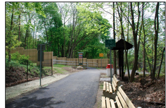
Above (top to bottom): View of Walden's "Little Lombard Street," which is the ADA compliant trailhead to the Walden-Walkkill Rail Trail at Woodruff Street; view of family enjoying a stroll along the rail trail; view of trailhead in Walden with benches.
