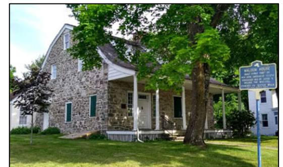
Above (top to bottom): View of Downtown mixed use buildings on Main Street; view of recently renovated Millspaugh Furniture on Main Street with new upper cornice and large display windows; and view of renovations which respect the character of the existing structure.
