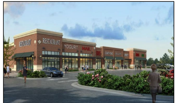
Above (top to bottom): Rite Aid built with design guidelines versus a Rite Aid built in a community without design guidelines; and a commercial plaza built with design guidelines which break up the mass of the structure and creates an inviting space.
